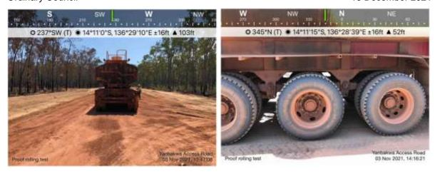
Proof rolling test with a water truck full of water: Package 6 CH. 24940 - 25986
